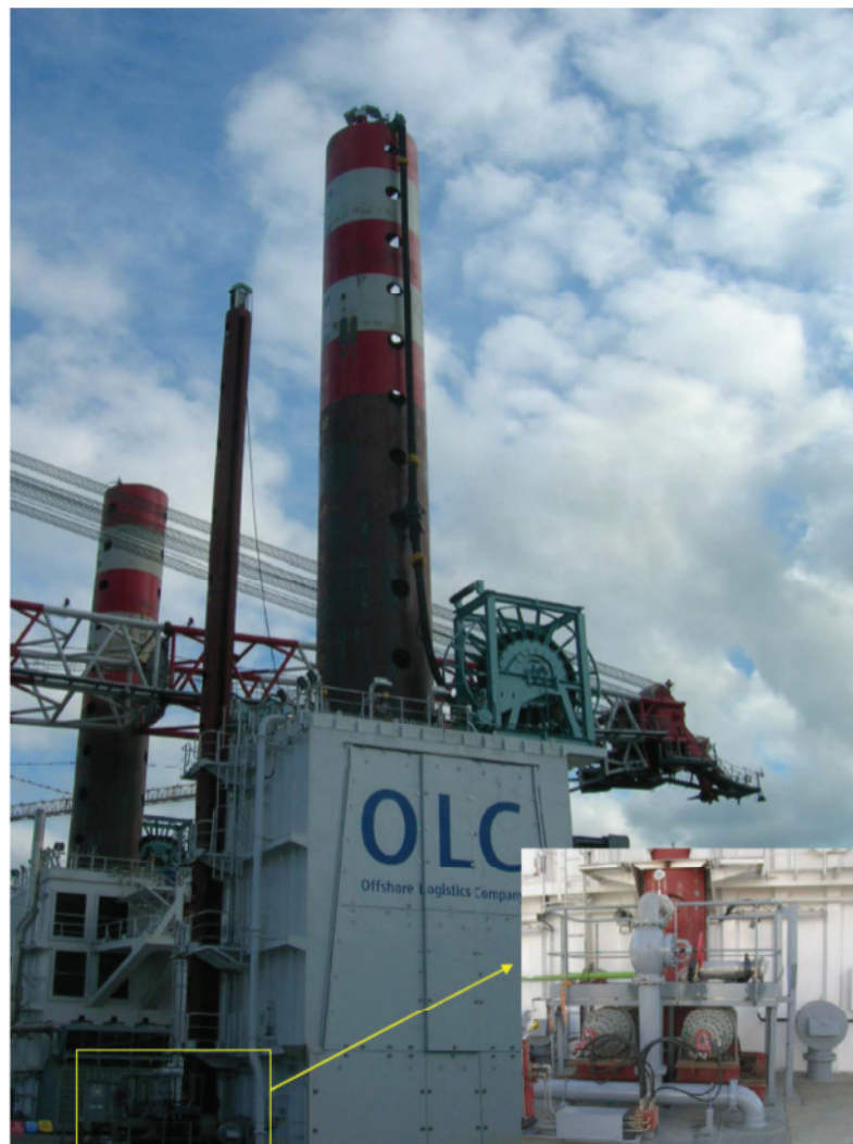
Figure 6-19 Suction Mast Location
